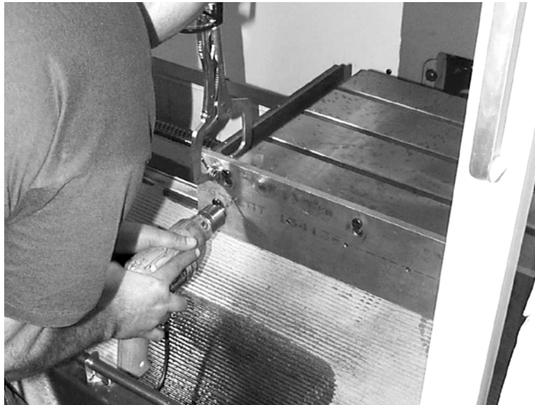
Figure 11-7 Drill Starting Holes
